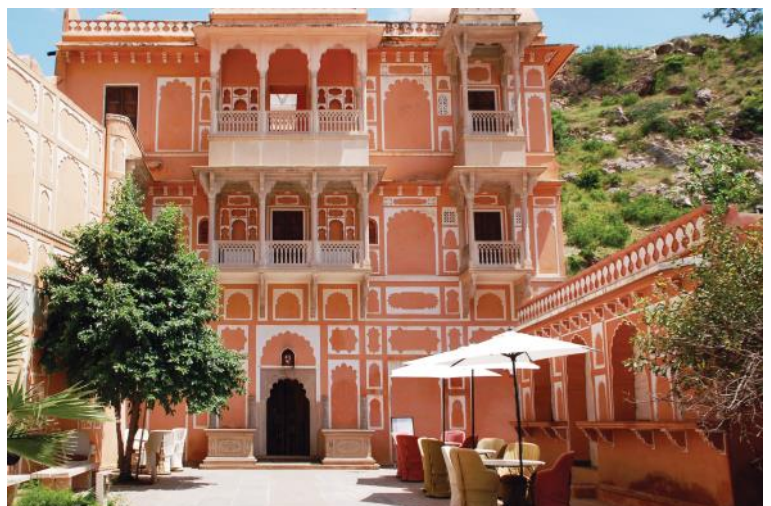
Figure 2. Facade and courtyard of renovated haveli, now the Anokhi Museum of Hand Printing (2006). Photo courtesy of Anokhi Archives.
